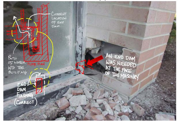
WATER WILL Get INTO THE SYSTEM THROUGH THE MORTAR JOINTS & FAILED SEALANT (OVER TIME)
